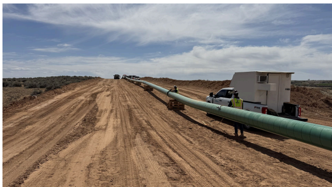
Radiography truck and darkroom on the right-of-way.
