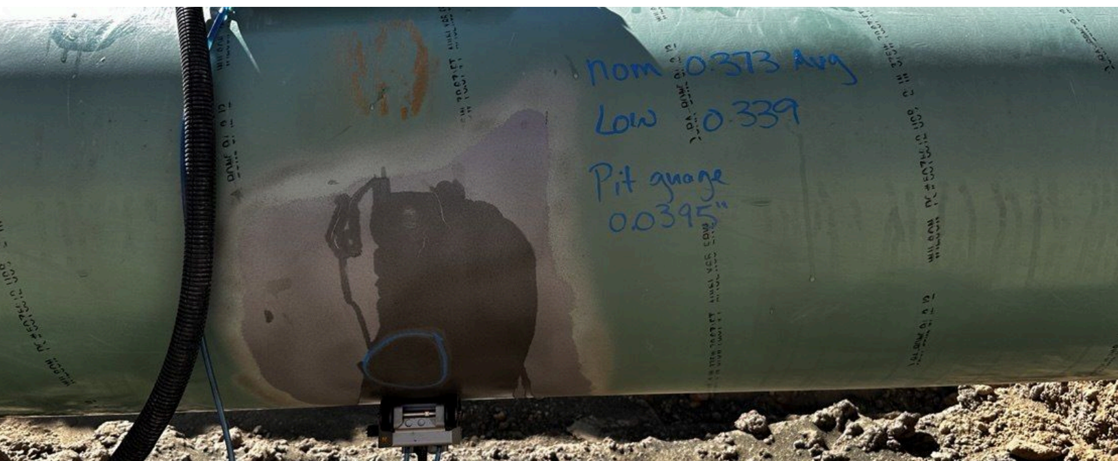
HydroFORM corrosion-mapping scanner on an integrity dig.
