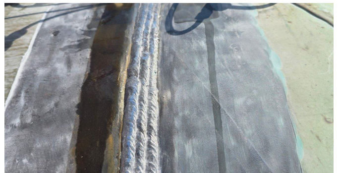
Encoded scanner and frame on a girth weld.
