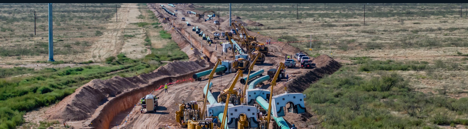
Mainline spread under construction — Prime Inspections crews work the weld as the spread moves, from mainline AUT through tie-in PAUT and repair.
