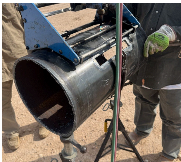
Cutting band mounted on a welder's test weld, with specimen coupons already cut out.
